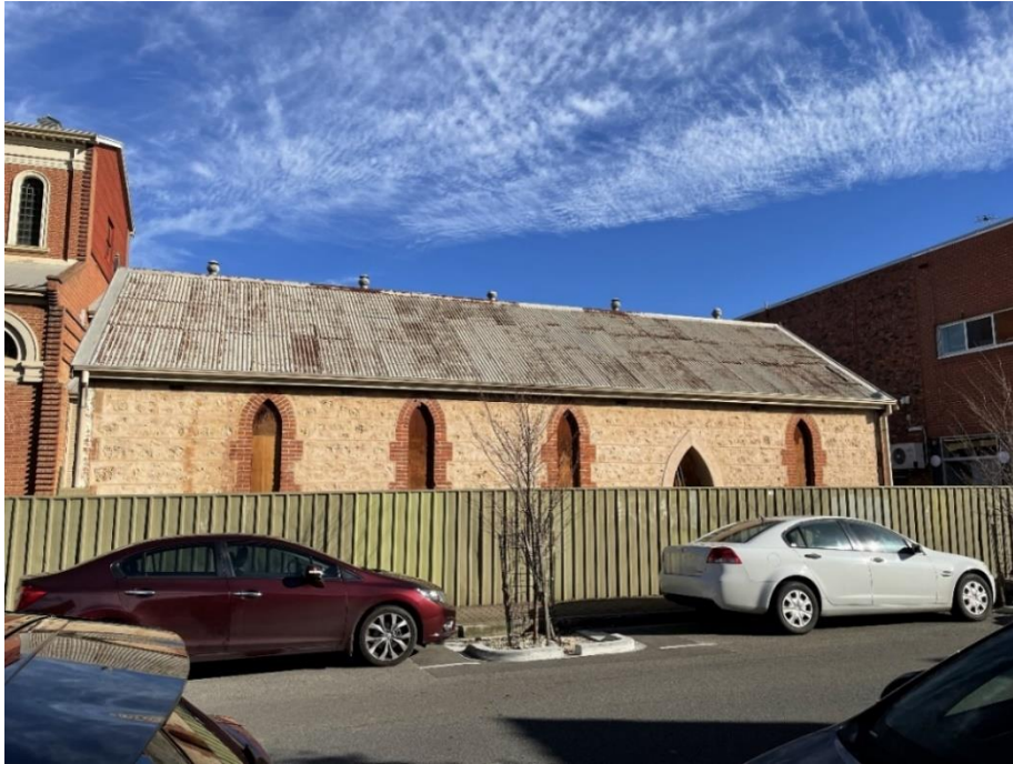
Eastern wall showing the original front entrance (on right) and windows with pointed arches and red-brick quoins.
