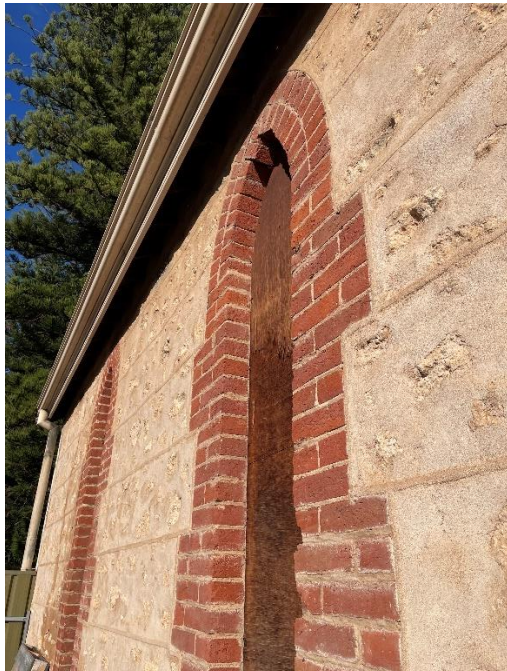
Repointing and repaired red-brick quoins on the eastern wall.
