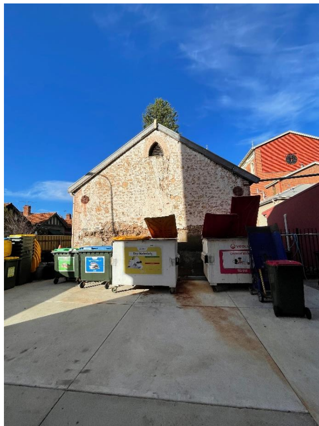
Northern wall of St Patrick's Schoolhouse.
