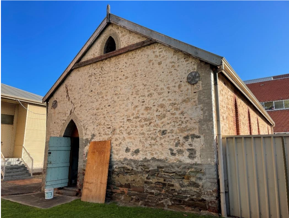
Southern wall of St Patrick's Schoolhouse showing one of the two doors, bluestone base courses, barge boards, finial and louvred vent with pointed-arch. Concrete rendering is visible in places including the quoins.
