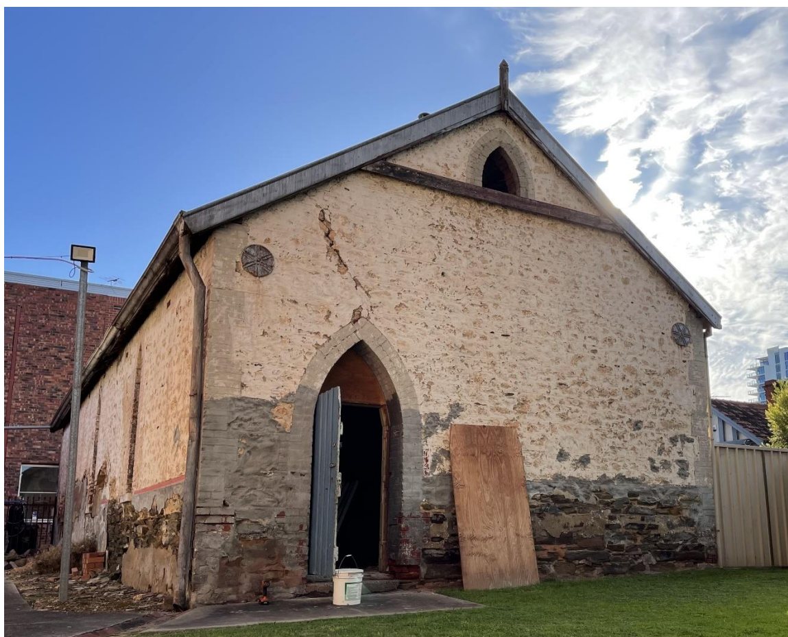
Southern wall of St Patrick's Schoolhouse.
