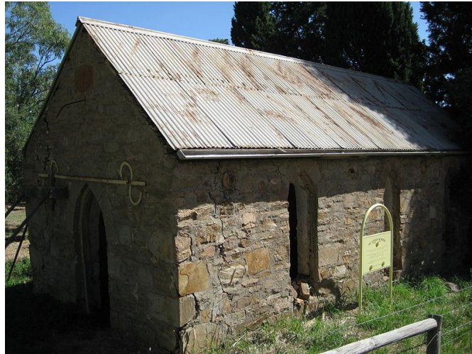
St. James School, Blakiston (LHP), prior to restoration and/or reconstruction, 2015.
