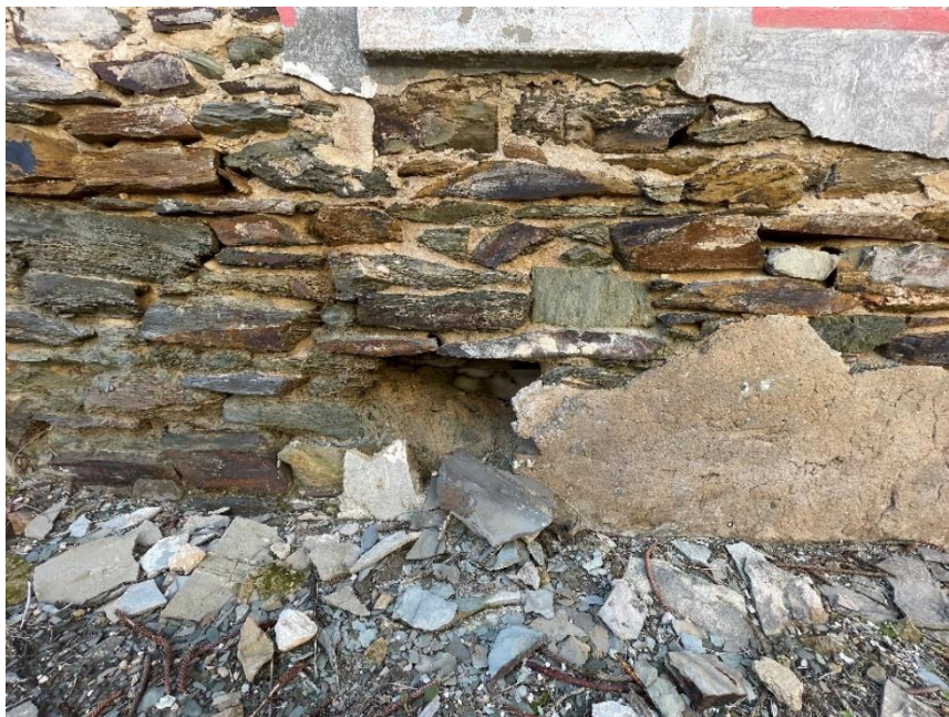
Bluestone base on the western wall showing where the building has been extended.
