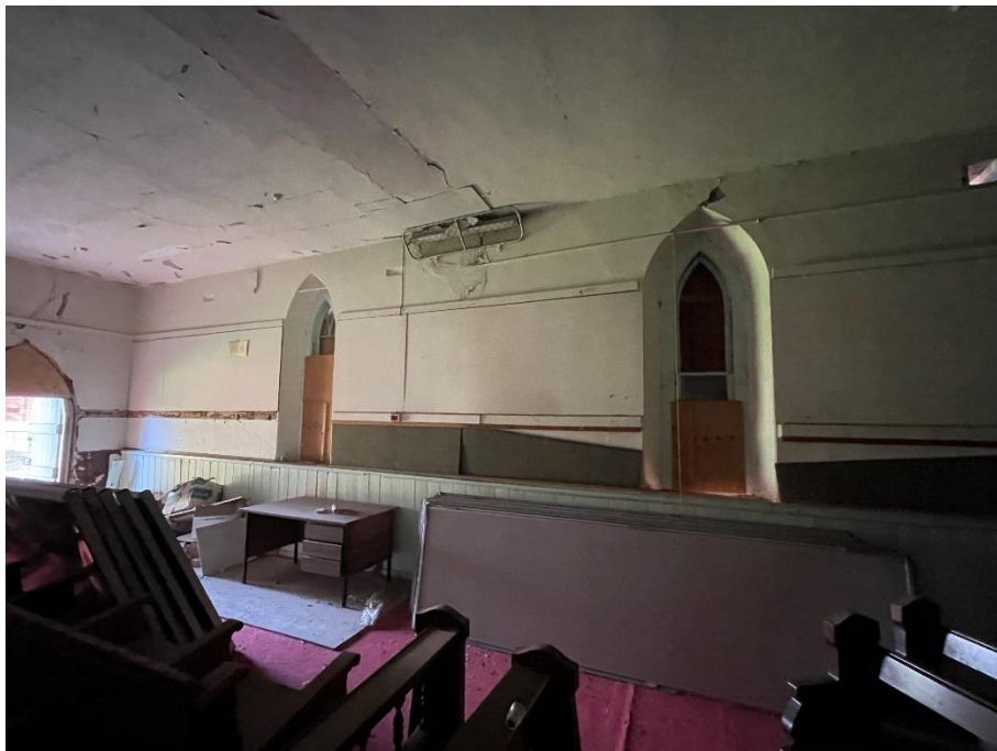
The interior side of the western wall showing two of three extant windows. The crack in the ceiling demarcates the original part of the building and the extended part.
