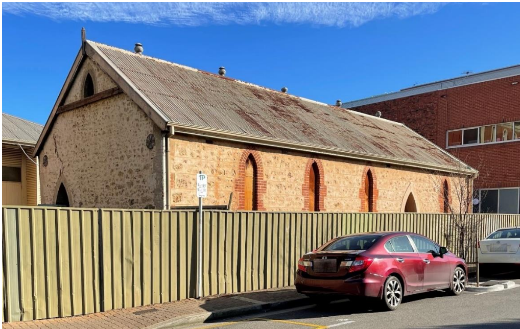
Eastern wall showing the repointed walls and repaired red-brick quoins.
