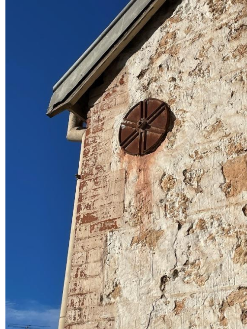
One of four cast-iron tie-plates
